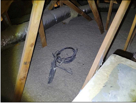
View of insulation
