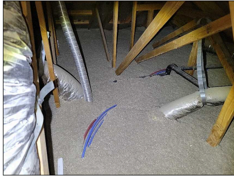
View of insulation
