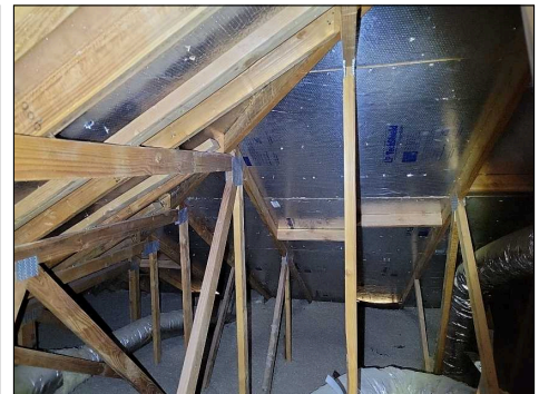
View of attic structure
