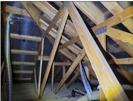
View of attic structure
