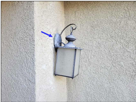
Fixture separating from the wall (pic 1) Fixture separating from the wall (pic 2) Outlet does not work. Missing gfci tab
