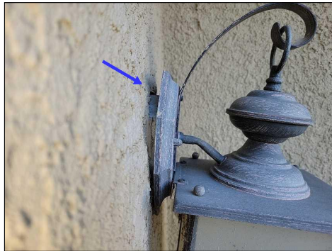
Fixture separating from the wall (pic 1) Fixture separating from the wall (pic 2) Outlet does not work. Missing gfci tab
