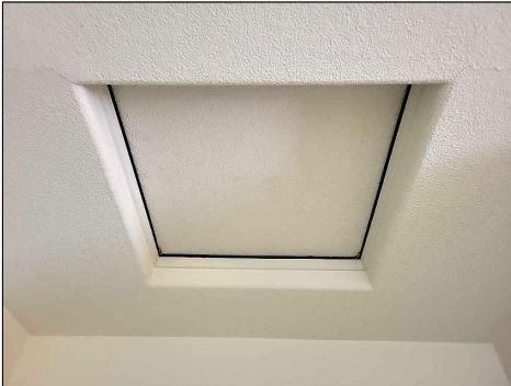
Access at up stairs hallway ceiling.
