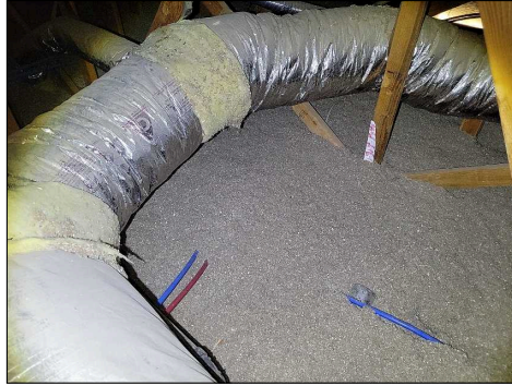
View of insulation
