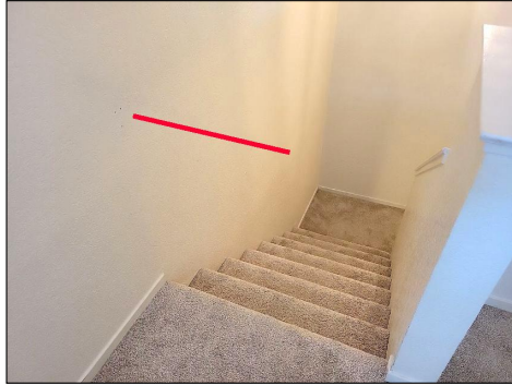
Missing handrail
