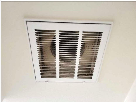
Filter is missing
