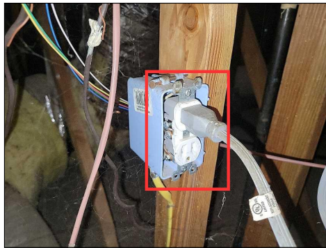
Outlet cover missing
