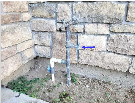
Main water shut off valve
