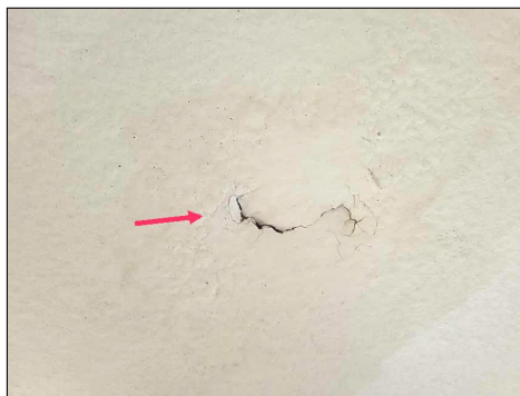
Past water damaged to ceiling in flex room
