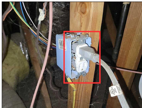
Outlet cover missing
