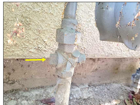
Main gas shut off valve
