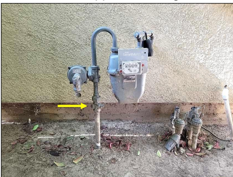
Main gas shut off valve
