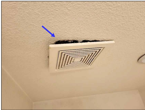
Up stairs bath fan is loose
