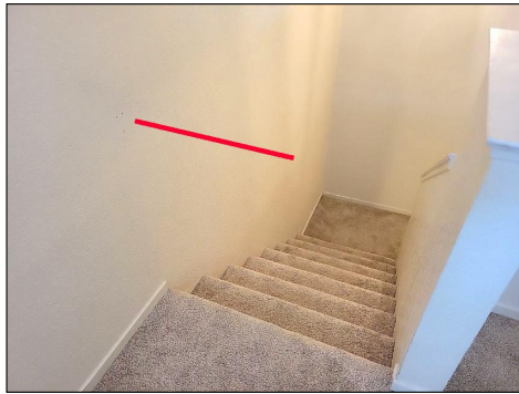
Missing handrail
