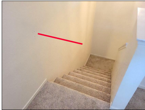
Missing handrail
