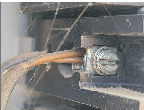
Double tap wiring
