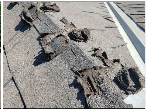
Roof damage
