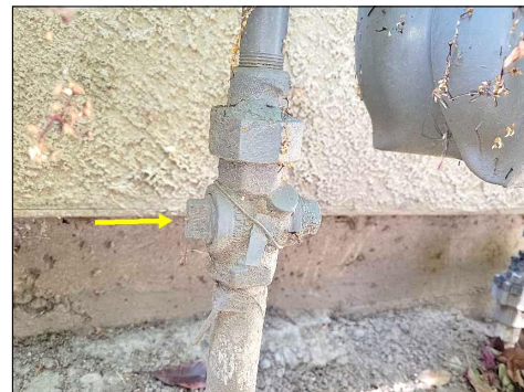
Main gas shut off valve
